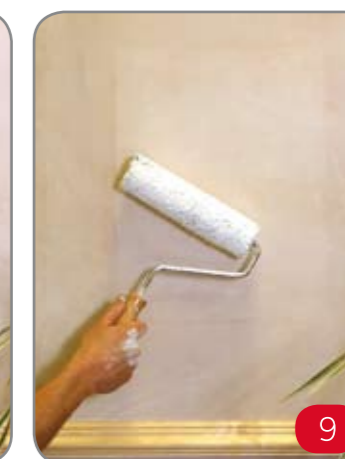
9 Allow plaster to dry thoroughly before using and before decorating with paint or wallpaper.
