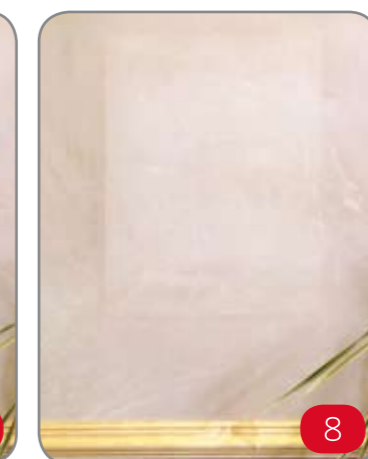
8 Skim with plaster (ordinary multifinish is fine). The best finish is produced when the entire wall is skimmed at the same time.
