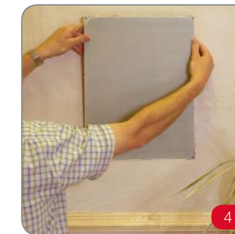
4 Position product in aperture. Connect loudspeaker to cable and test its operation.
